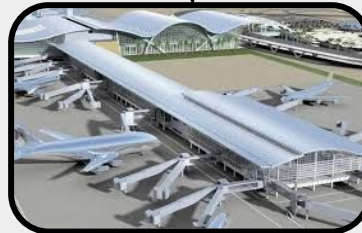
Dholera International Airport
