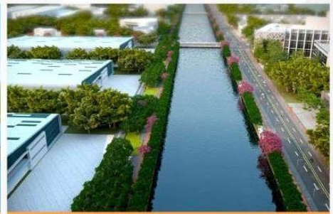
Water Side Area
